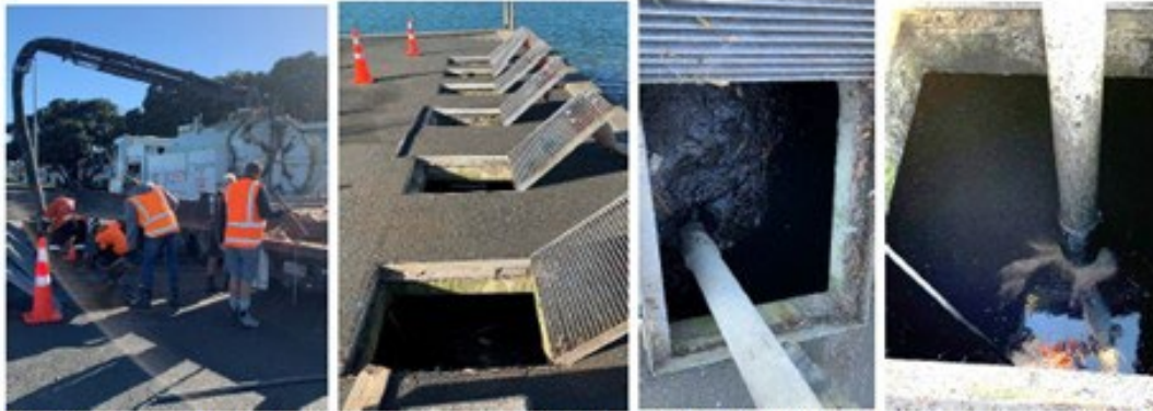
Above: Southey's. Then: the six tanks, nearest 3 for solids settlement. Above: sludge tank full. Right: tank now empty.
