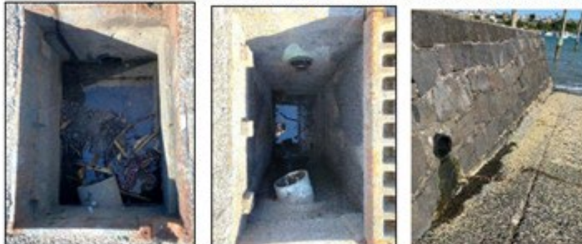
Left: one of the three grated drains which flow into the settlement tanks, full of debris. Centre: the same drain, now empty, showing its depth. All three were cleared. Right: cleaned and filtered water flowing down ramp.
