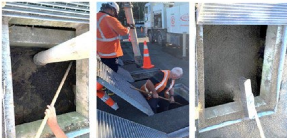
Left: dark contaminated sand being sucked out and removed. Centre: Each sand tank raked to ensure full coverage of new sand. Tanks extend well under asphalt. Right: Dirty sand was replaced with 3 cubic metres of clean sand.
